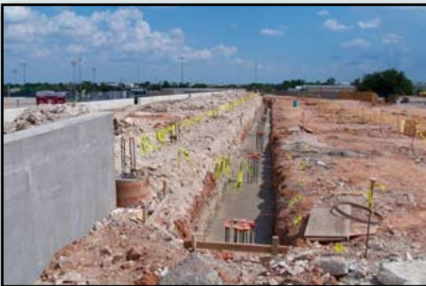
Upper-Seating Grade Beams
