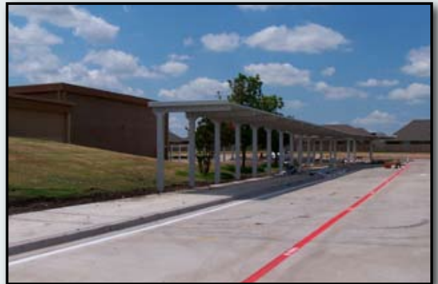
Covered Walk-Way at Hewitt Elementary
