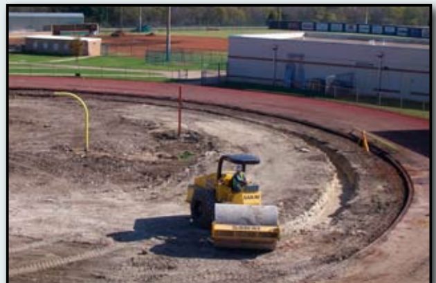
Preparation for New Field Surface
