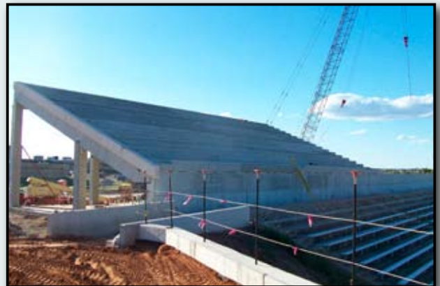
Grandstand View from Field Side
