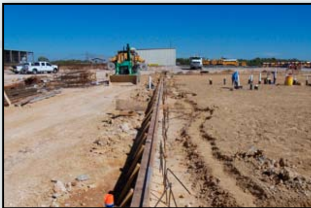
Concrete Paving for Bus Drive
