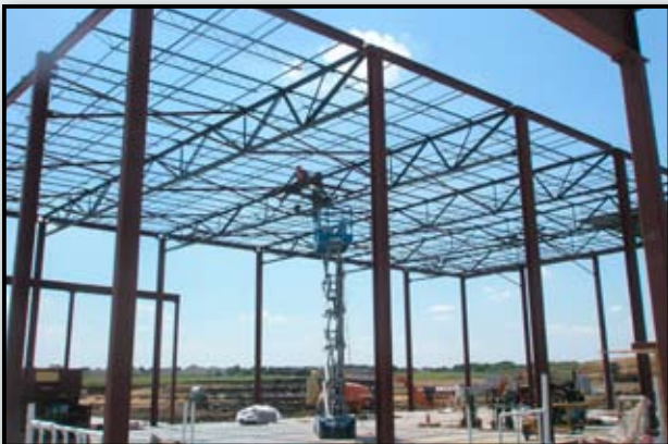
Steel Erection at Gymnasium Area
