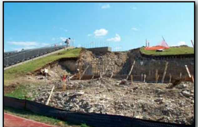
Home Side Retaining Wall
