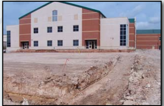
High School Foundation Work
